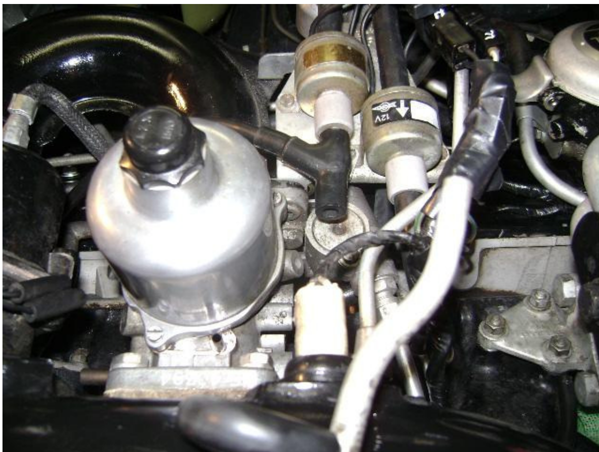
The finished installation waiting the fitting of the vacuum pipe
