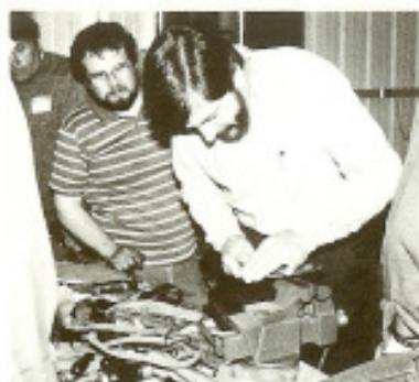
Above: To correct uneven wear, Ralph Curzon files the servo lining in a circular pattern, always touching two sides of the plate at once. Left: Ken Collier, FL, gives it a try.
