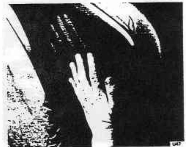
Fig. S17-13 Finger furrowing — an incorrect method of flatting
